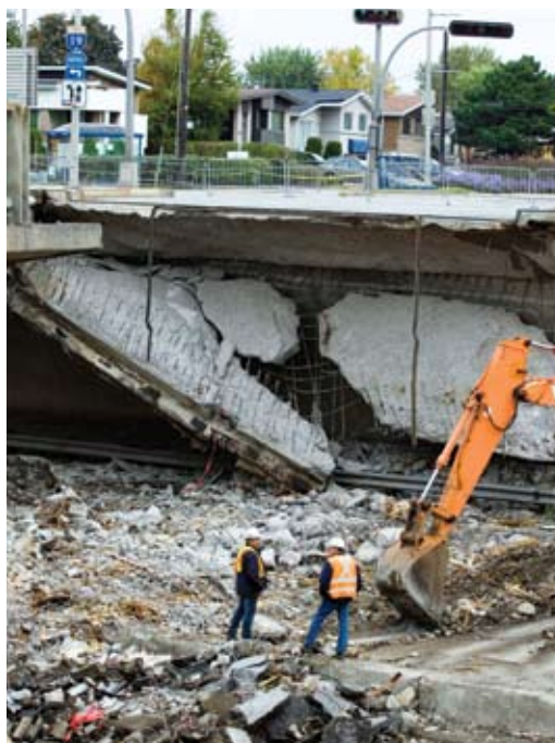
Rebuilding an overpass that collapsed in Laval, Quebec, in 2006 took money as well as muscle. Canada’s cities face shortages of funds for replacing major parts of their aging infrastructure.
